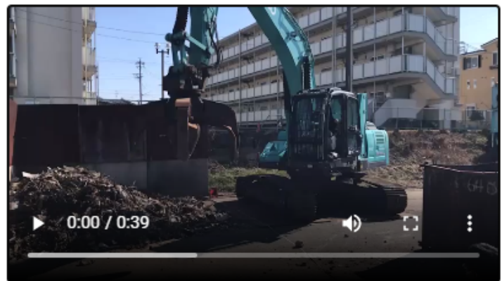
Automatic recognition and transportation of material for recycle (2x speed)
