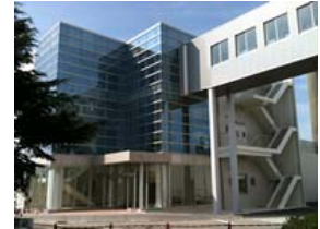
Fig.1: The new EIIRIS building.
